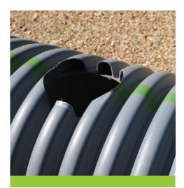
Core a hole perpendicular to the host pipe using the recommended hole saw. Remove the coupon from the saw. Deburr the cored hole.
