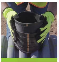
Use the coupon to estimate the separation between the two sleeves and fit the two sleeves together. Be sure the gold lines on the sleeves are lined up.
