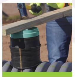
Drive the plastic hub into the rubber sleeves with a 4 lb. mallet and block of wood. Stop when the rubber sleeve meets the red line.
