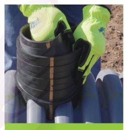
Insert the rubber sleeves into the cored hole, with the gold lines perpendicular to the pipe. Once in place, pull up on the inner sleeve and push down on the outer sleeve until fitted to the hose pipe.
