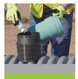
Apply soap solution to inside of the inner sleeve and on the PVC hub. Insert the PVC hub into the sleeve by hand until snug fit, aligning the red line on the hub with the gold lines on the rubber sleeves.
