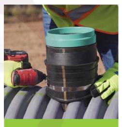
Place and tighten the stainless-steel band.
