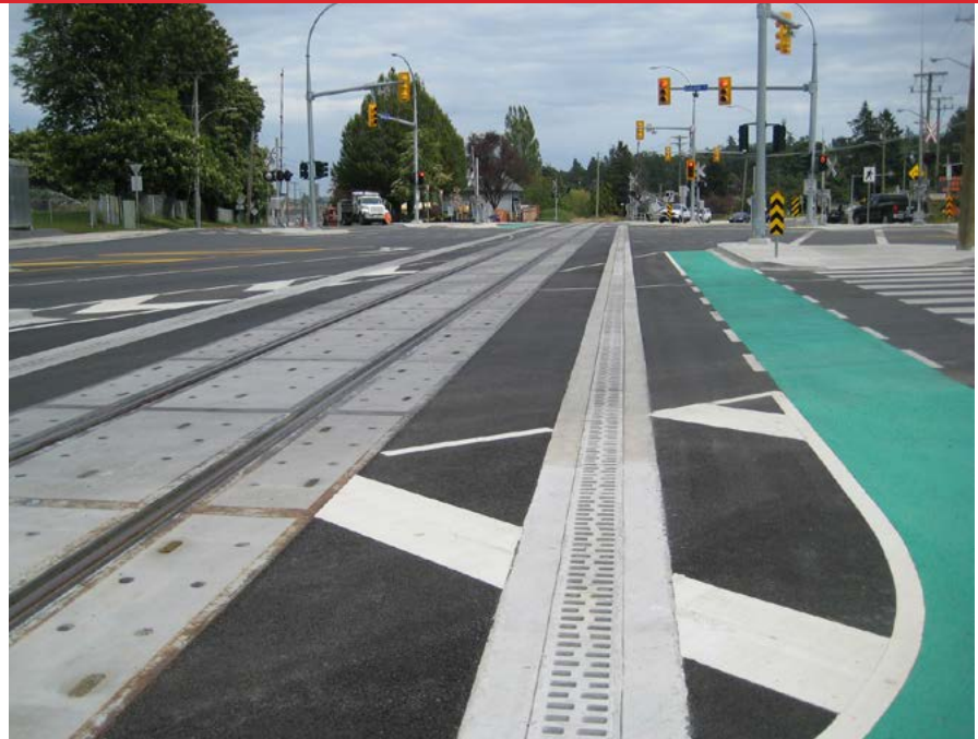
Monolithic polymer concrete 8" trench drain with high capacity intake slots and pipe connection flume.
